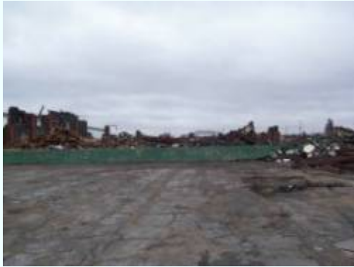
Phase Nine Demolition at Quonset
