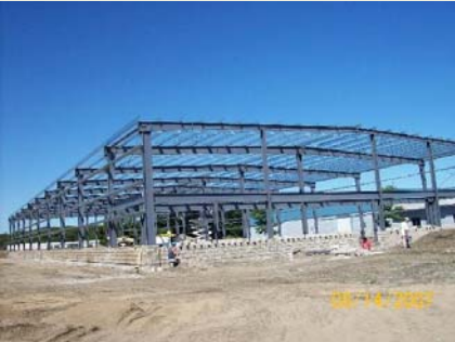
Flurry of Construction as Quonset
