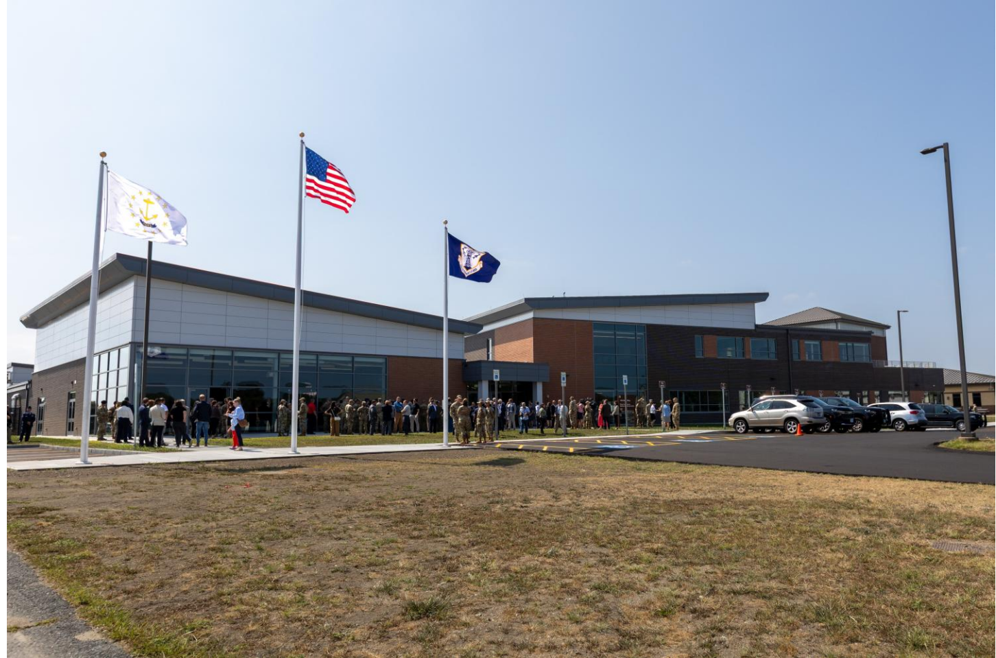
Headquarters, Dining Facility & Medical Facility Building
